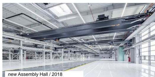
new Assembly Hall / 2018
