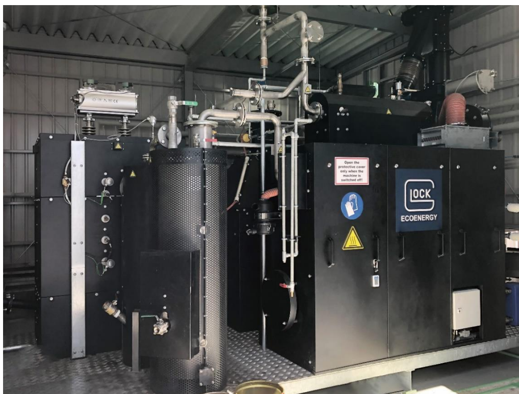
Wood gas combined heat and power plant by GLOCK ecotech GmbH
