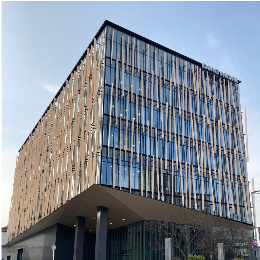
Outside view of Nara PDC under construction Design by Kengo Kuma and Associates
