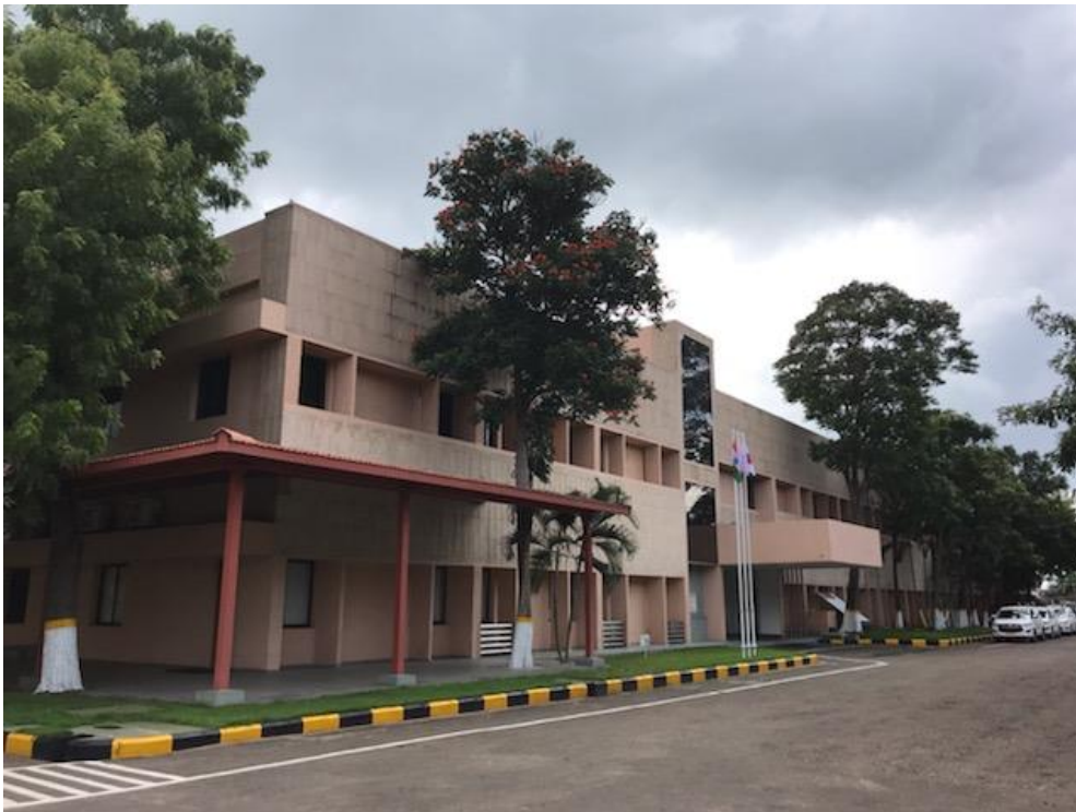
Lakshmi Machine Works Limited (Exterior)
