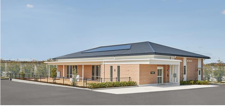
Exterior of the facility in Iga Campus
