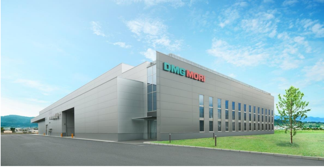
Exterior of System Solution Plant
