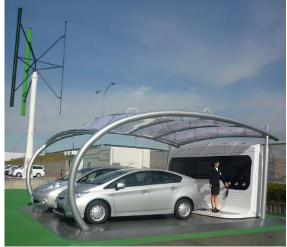
From left: Wind power generator (WindCarrier) Redox flow battery (CellCube) Power charge station (E-filling station)
