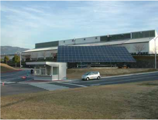
The photovoltaic system installed at the Iga Campus
