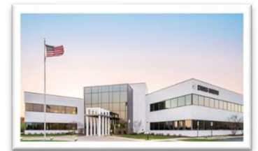
DMG MORI Federal Services office
