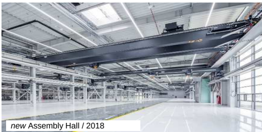
new Assembly Hall / 2018
