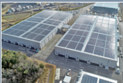
Self-consumption solar power generation system
