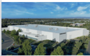
Davis CA factory
